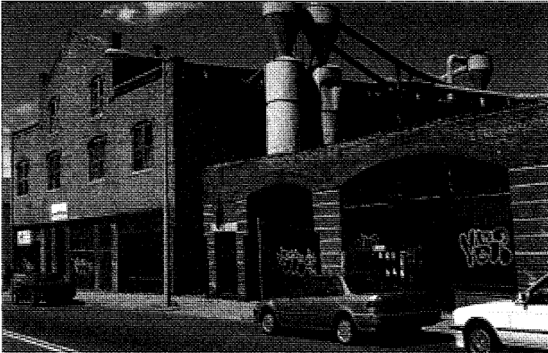
Site for Youth Build Cabinet Shop
