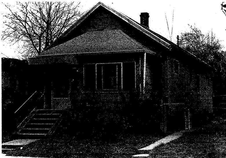
West Clinton home before renovation.
