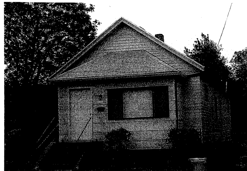
West Clinton home after renovation by REACH.
