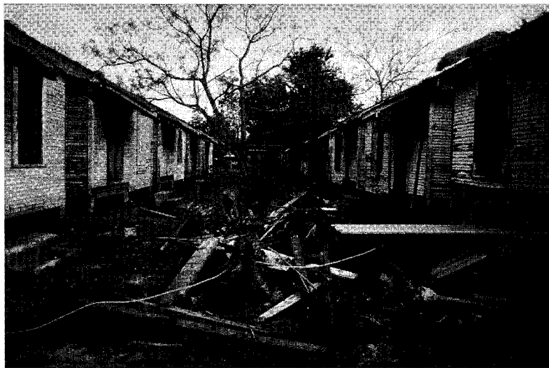
Interior courtyard at Project Row Houses before renovation.
