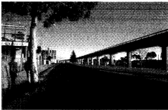
BART track behind Hismert Hin-nu
